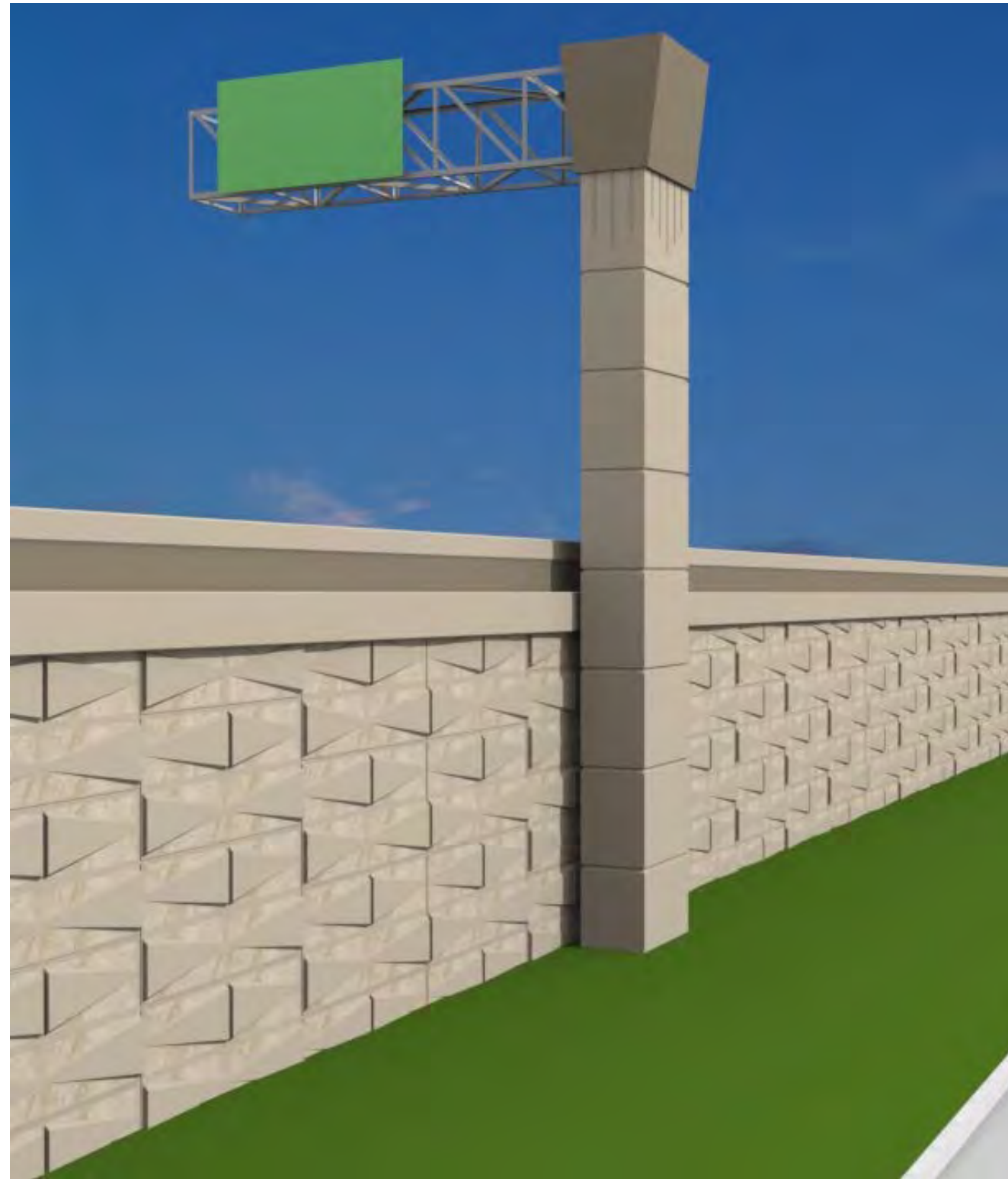
Major Guide Sign / ITS Support Structure
